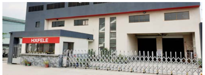
Häfele Production Plant Binh Duong, Vietnam
