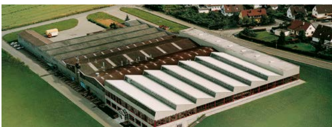
Häfele Production Plant Jettingen, Germany
